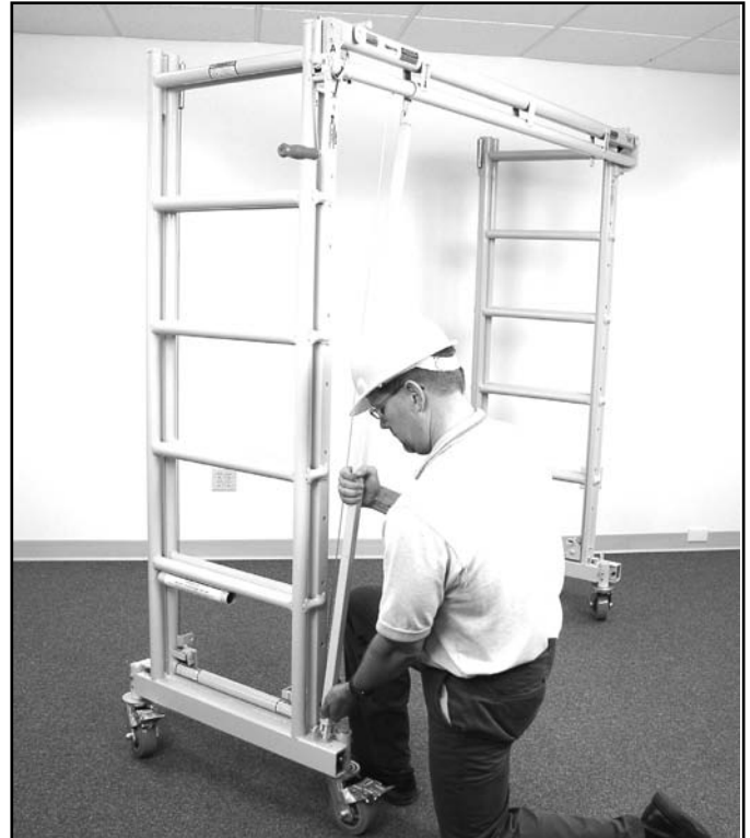
7) Jog base of end sections to facilitate brace pin alignment. DO NOT hammer on braces.
