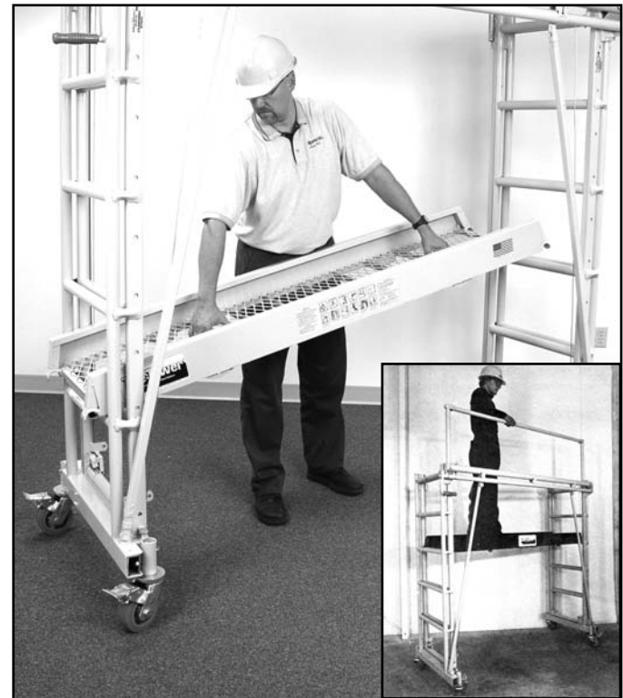
8) For platform heights from 2' to 6', the deck may be placed on lower rungs. For added safety use guard rails even when deck in on lower rungs.
